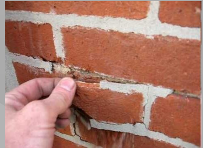
Using of cement with old bricks
