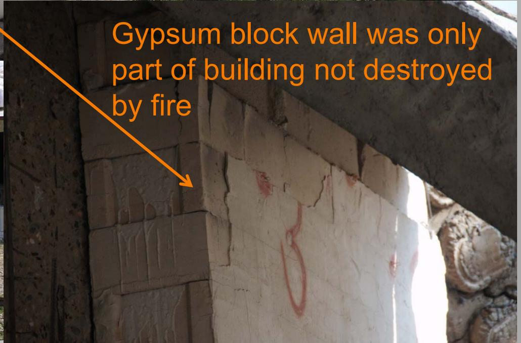
Gypsum block wall was only part of building not destroyed by fire
