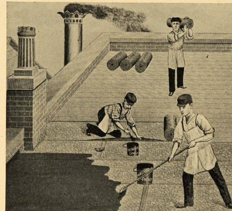
Below is pictured workmen in the process of laying CAREY'S MAGNESIA FLEXIBLE CEMENT ROOFING.
