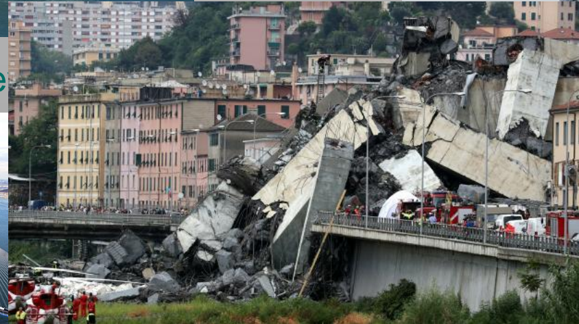
Morandi Bridge, Genoa
