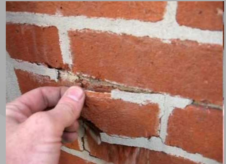
Using of cement with old bricks
