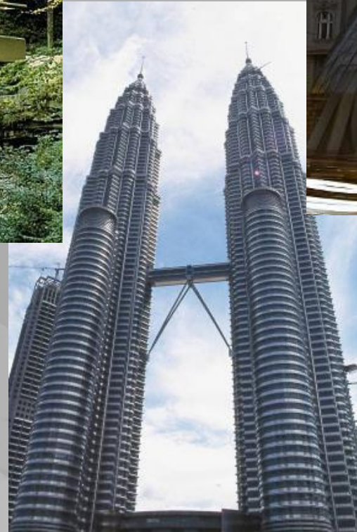
Petronas Twin Towers, Kuala Lumpur César Antonio Pelli, 1999
