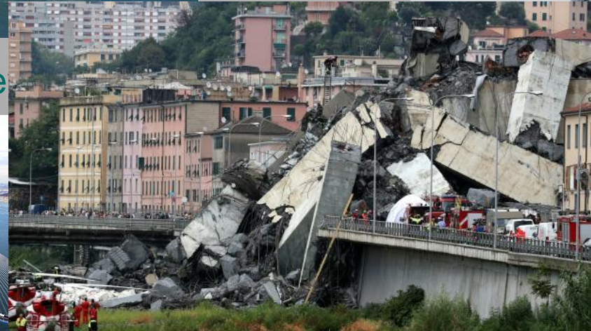
Morandi Bridge, Genoa
