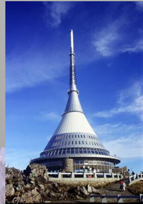
transmission tower Ještěd, CR
