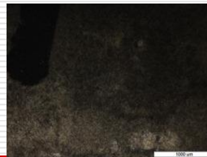
(a) After 7 days corrosion
